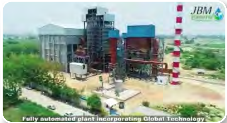
Fully automated plant incorporating Global Technology
